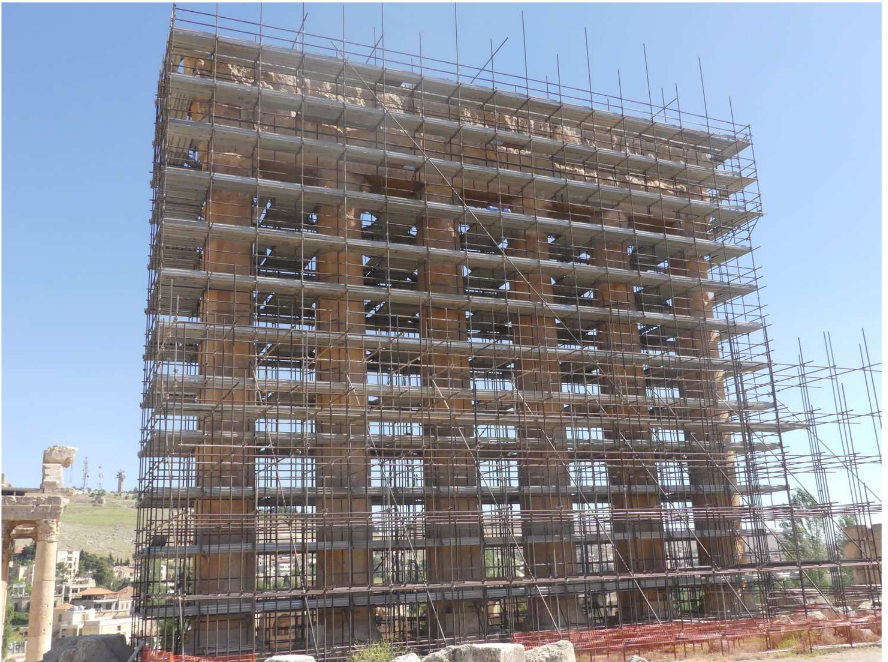
Restoration of some of the columns of the Temple of Jupiter.
