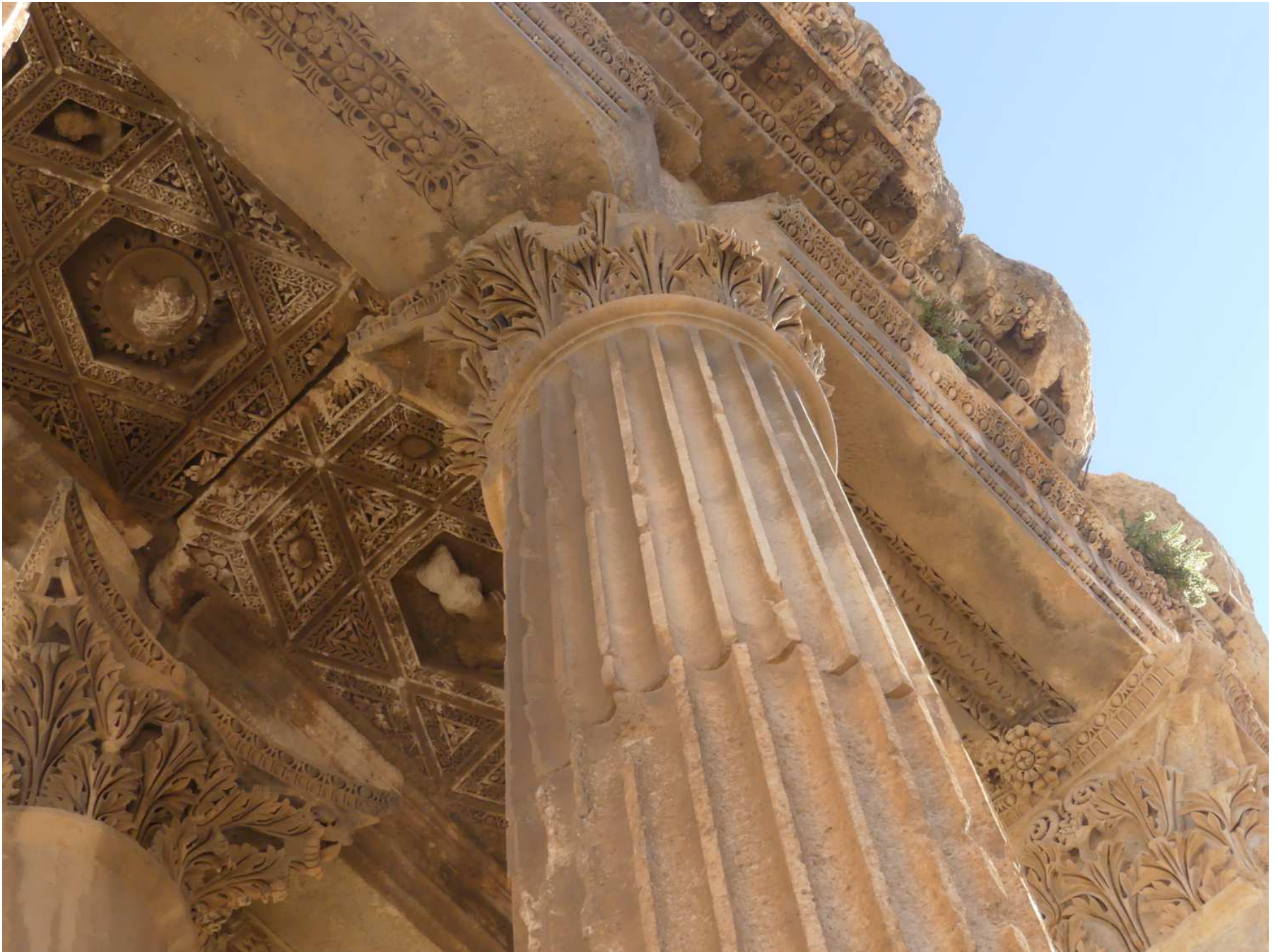
Looking up at the ceiling of the outer structure.
